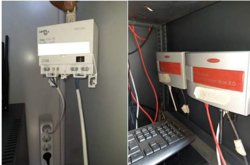
Fig. 22. Installation of the ripple signal receiver to the smart logger.
