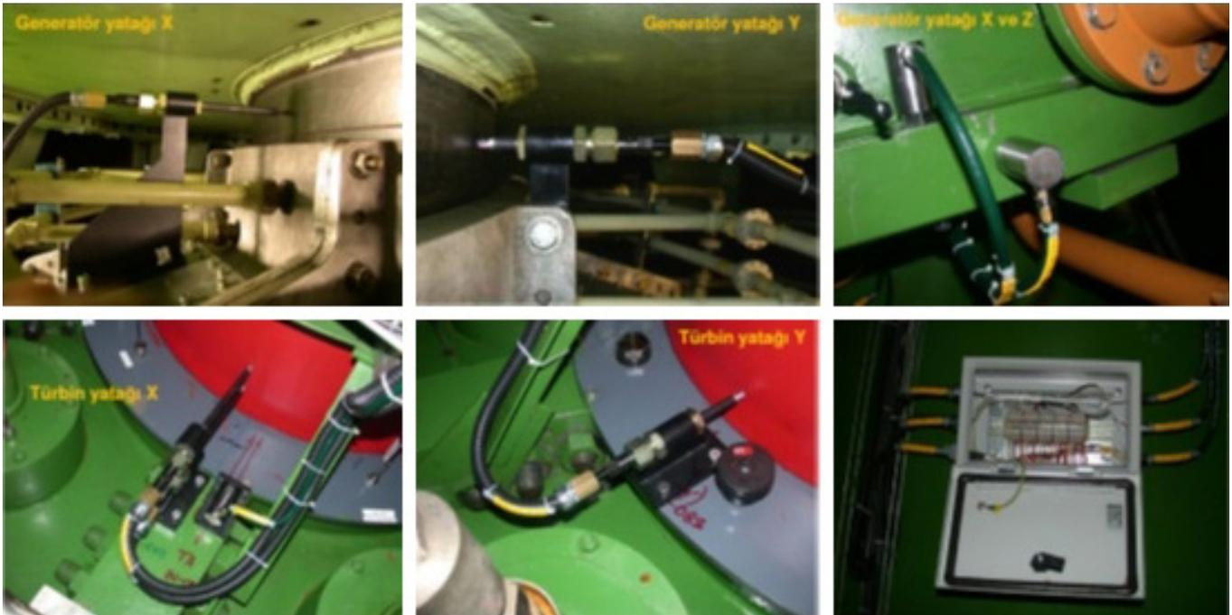
**Figure 13.** Placement of the sensors used in generator and turbine bearings
